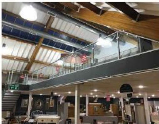
(Photo 2) at first floor level looking at 2nd floor mezzanine
